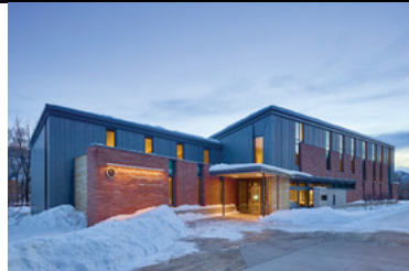
ARCHITECT The Rocky Mountain Institute's New HQ Has No Central Heat or A/C
